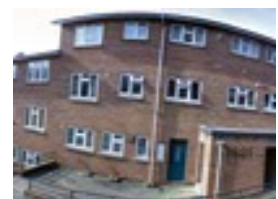
Figure 22: A typical purpose built 2-bed flat, 1945-1980
